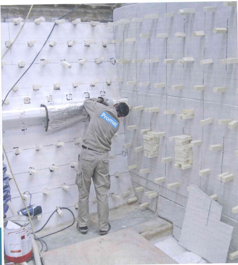
Promat's Promaguard A240 Plus can achieve in excess of four hours' insulation in the event of fire, without affecting weight and space saving criteria
